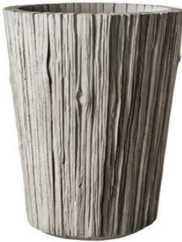
Rough textures were created with sandblasted cedar forms.
